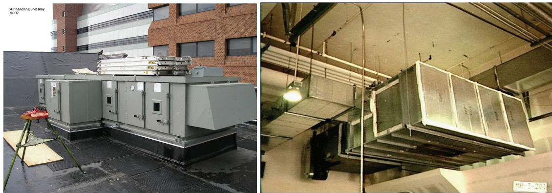
Figure 1. Roof mounted and rod hung air handling units
